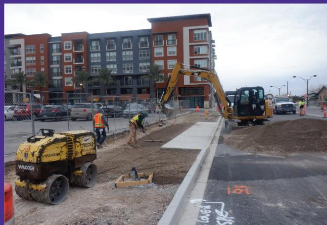
Crews grading for the sidewalk behind a new concrete driveway on Carson Ave.
