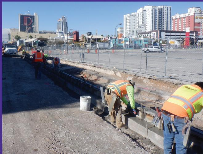
**Crews placing concrete forms for the new curb along Carson Ave, between 8th St and 9th St.**
