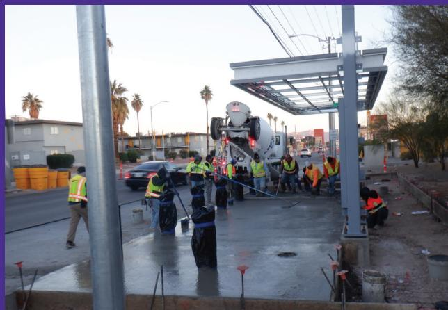
**Crews pouring and finishing the concrete for a new passenger shelter on Maryland Pkwy near Reno Ave.**
