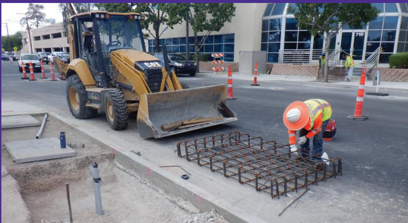
Concrete will be poured around this rebar cage to form the footing for a new streetlight.
