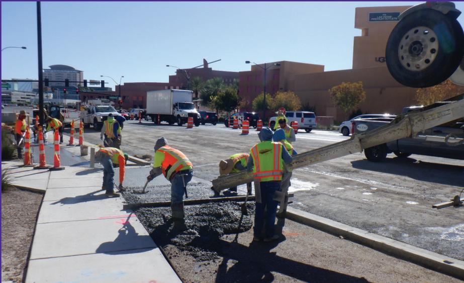
Crews pouring concrete and smoothing/finishing the surface for a new 10-foot sidewalk along Bonneville Ave, just east of I-15.
