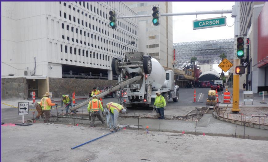
Crews pouring concrete for a valley gutter on Carson Ave at 3rd St. Valley gutters at cross streets are often built in halves to maintain access for businesses in the area.
