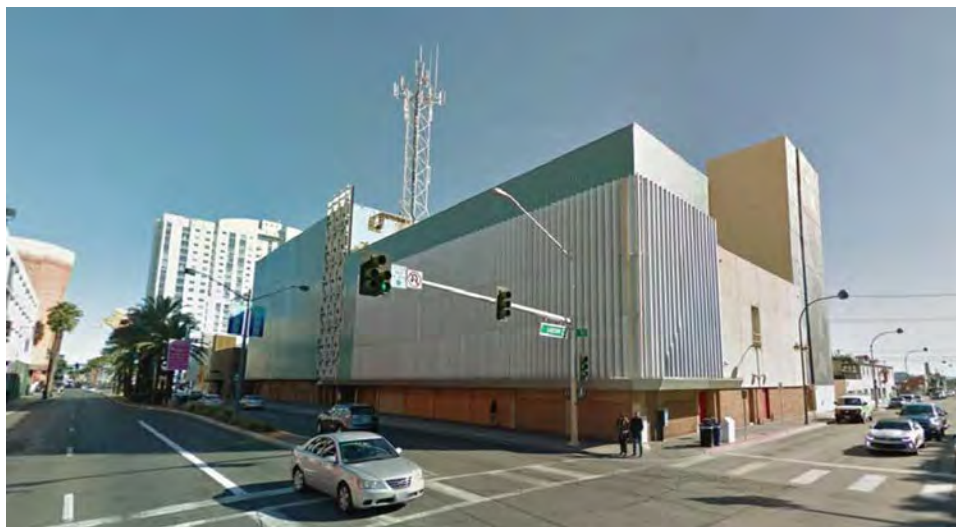
Central Telephone Building, facing northeast
