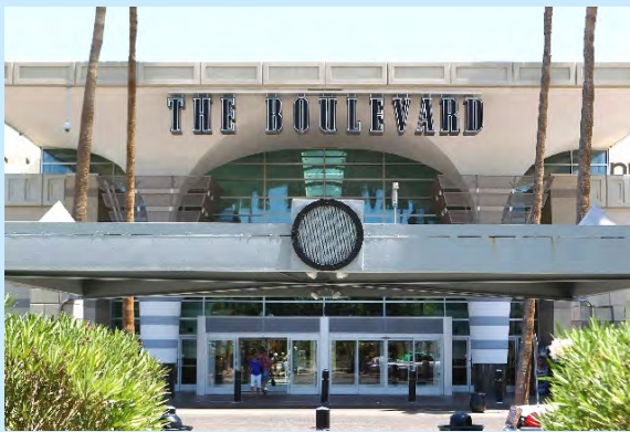
The Boulevard Mall
